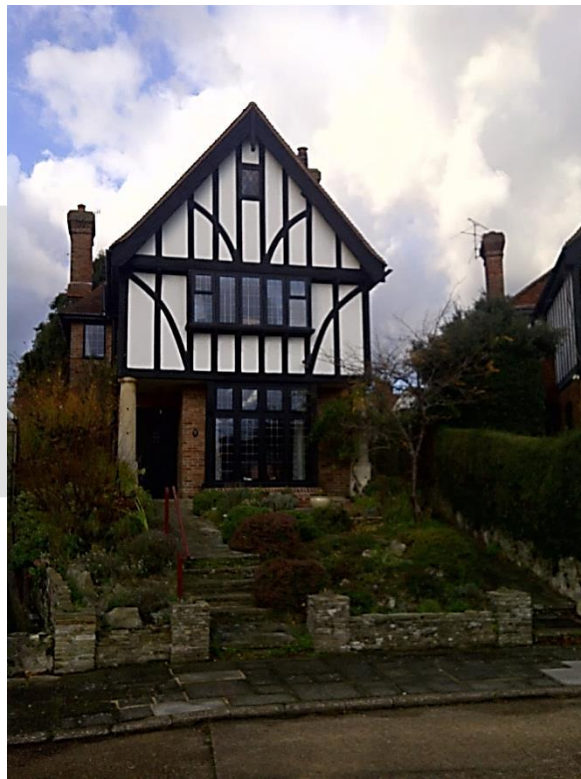
The Park Close – Subject to an Article 4 Direction and a designated Conservation Area
